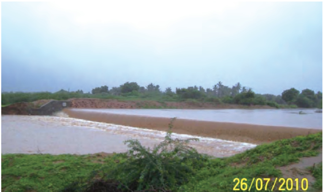
Over flowing check dam in basin area
