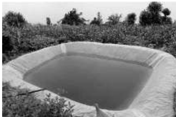
Rainwater Harvesting System
