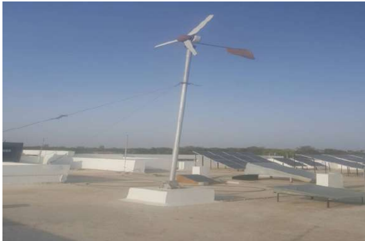
Figure : 5kW Hybrid Solar Wind Power System at College of Agricultural Engineering and Technology, Anand Agricultural University, Godhra
