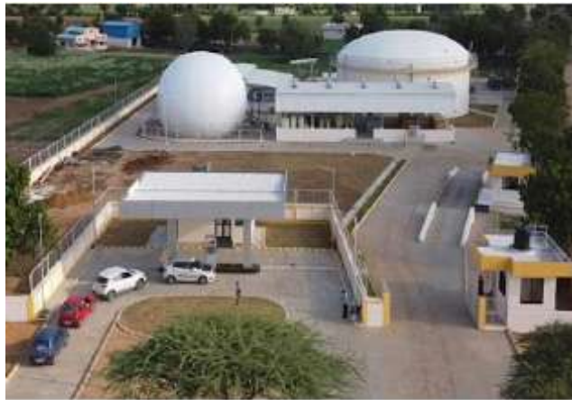
Fig.9: Bio-CNG plant of Banas Dairy
