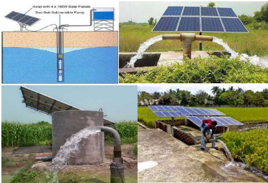
Figure : Picture of Solar Pumping Systems on Field
