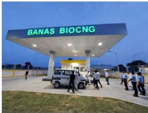
Fig.15: Bio-CNG Filling Station
